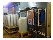
To reduce overall energy use and production costs, Con-Serv came to the rescue with a specially designed RO System to dewater the maple sap prior to boiling. With Con-Serv system in place, owner Bill Henry, says "that he can remove at least 75% of the water from the maple sap without affecting the quality, or taste, of the finished product". Actually "it's better" he says "as the finished product comes out a little lighter in color".
